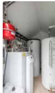
Heating The hot water cylinder and boiler operate in conjunction with a ground source heat pump. It is housed in a purpose-built shed.
